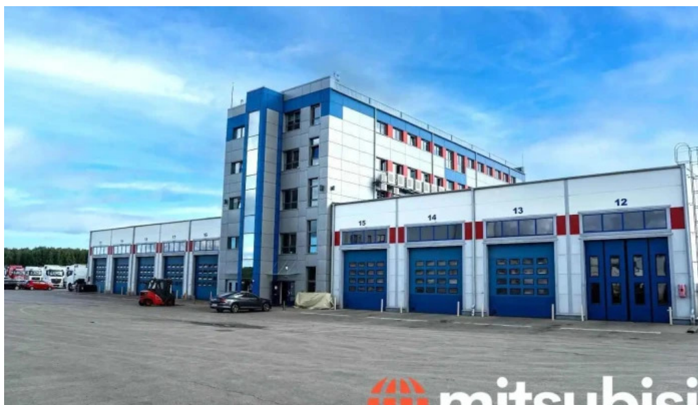
Zk 9 truck and trailer service mērupe
